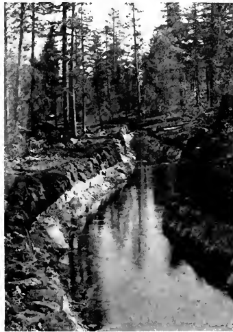
FIG. 2.—VIEW OF MAIN DITCH.
